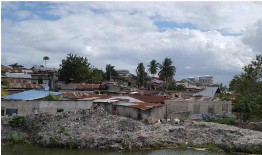
Figure 3: Some of the structures at site
